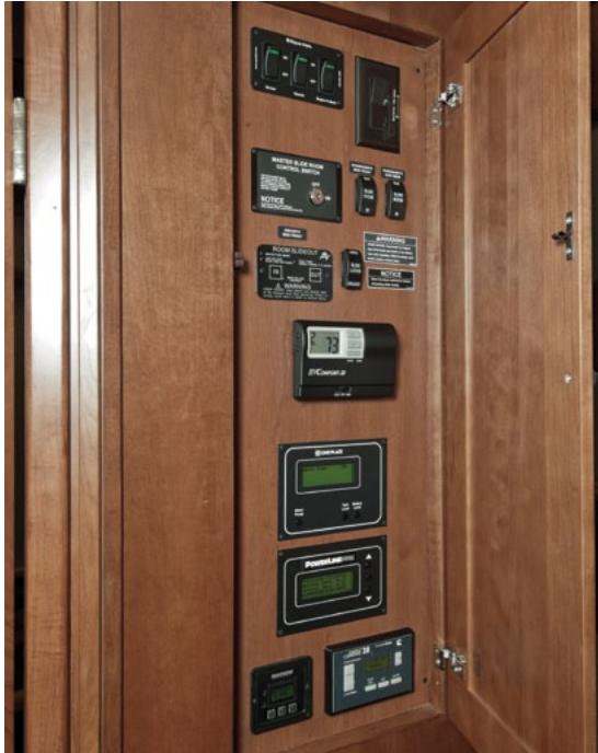
The PowerLine® Energy Management System , which minimizes tripped campground circuits in periods of high demand, is part of the OnePlace® Systems Center which places frequently used controls in one convenient location.
