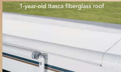
1-year-old Itasca fiberglass roof
