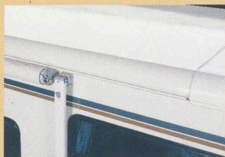
1-YEAR OLD ITASCA FIBERGLASS ROOF
