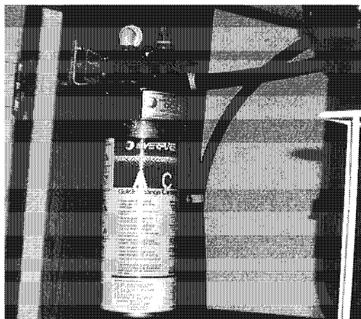
Water Filter Assembly - Below Galley Sink
