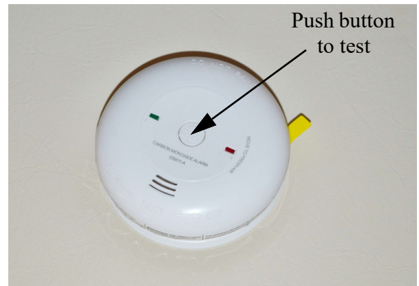
Carbon Monoxide Alarm
