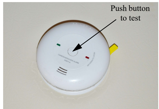
Carbon Monoxide Alarm
