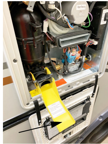
Water heater Easy Drain Lever in lowered position. -Typical View
