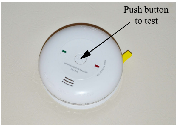
Carbon Monoxide Alarm
