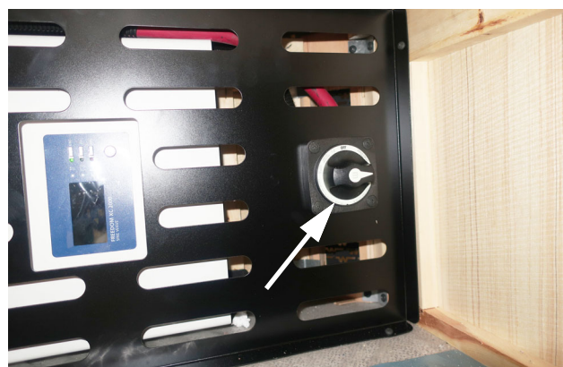
Inverter/charger disconnect switch. (Located inside the passenger's side compartment door next to the inverter). -Typical View
