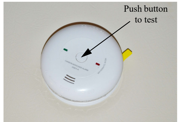
Carbon Monoxide Alarm
