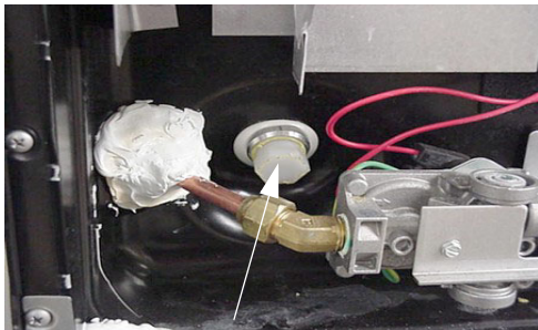
Water Heater Drain Plug (Remove with socket)
