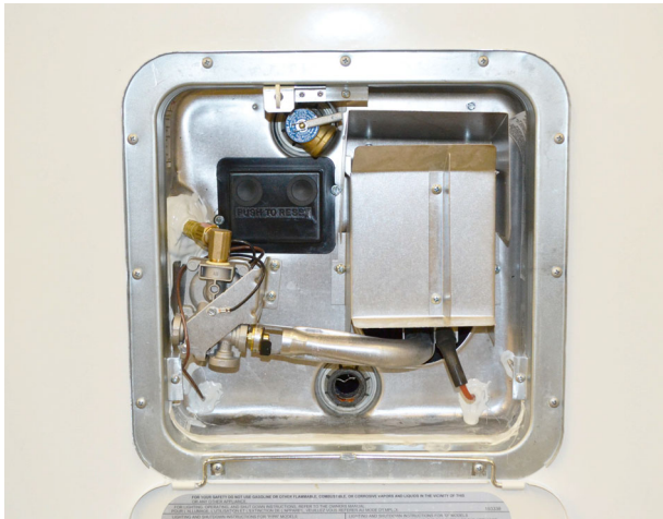
Water Heater Exterior Service Access
