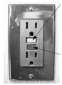
GFCI Outlet (Ground Fault Protector)
