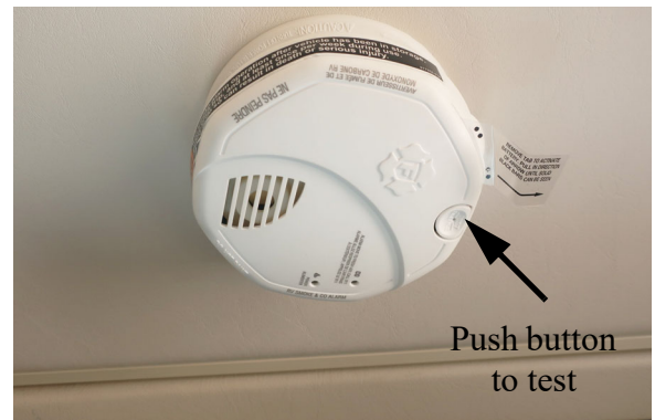
Smoke/carbon monoxide alarm. -Typical View
