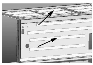
A cut away drawing with the back wall removed. The brackets run horizontal on the inside wall and on the ceiling. These are not visible. Locate these brackets using a magnet.
