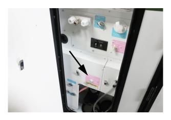
Waterlines Valve #3 Located on Water Service Center. -Typical View
