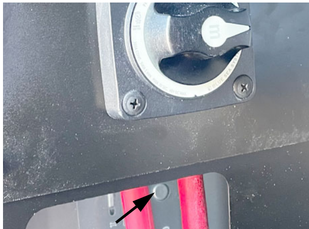
Ensure that the inverter box power button is pushed in for the monitor panel to be able to operate the inverter. -Typical View
