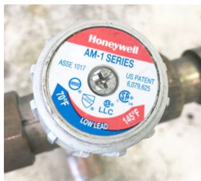
Hydronic Heating System Tempering Valve (Located below dinette seat - remove screws and panel to access)
