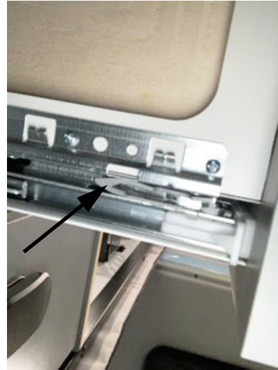
Reach under each side and pull gray tab outward to remove drawer from guide. -Typical View
