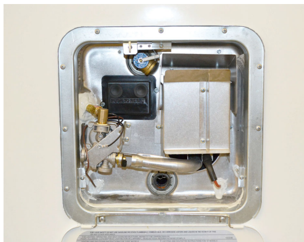
Water Heater Exterior Service Access
