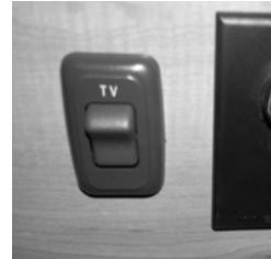
Master 12V Power Switch (Located on underside of cabinet near TV)
