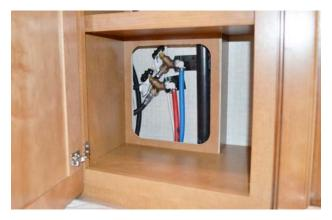
Water Supply Faucets (Located inside cabinet front of washer/dryer remove access panel)
