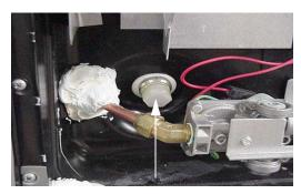
Water Heater Drain Plug (Remove with socket)
