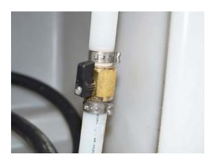
Water Tank Drain Valve -Typical installation shown
