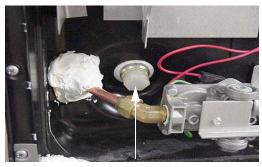
Water Heater Drain Plug (Remove with socket)
