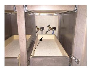
Water Supply Faucets (Located inside pantry cabinet above washer/ dryer, remove panel to access)
