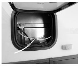
Ice Maker Drain Line (Located in exterior Residential Refrigerator service compartment)
