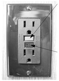
GFCI Outlet (Ground Fault Protector)
