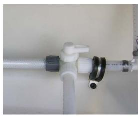
Waterline Drain Valve -Typical installation shown
