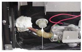
Water Heater Drain Plug (Remove with socket)
