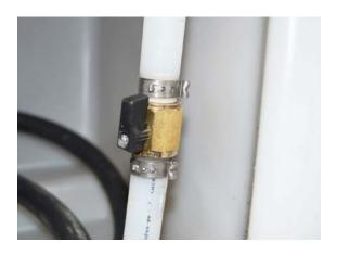
Water Tank Drain Valve -Typical installation shown
