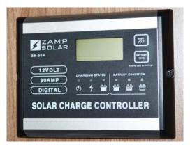
Solar Charge Controller (Located near monitor panel)
