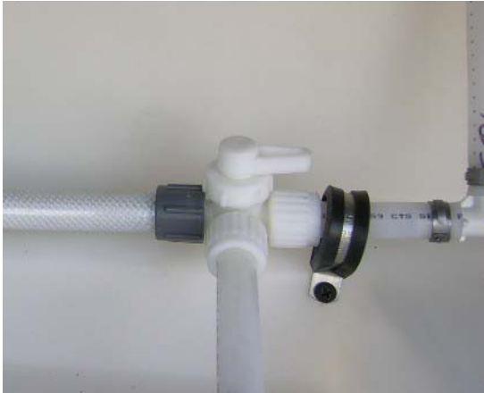
Waterline Drain Valve -Typical installation shown
