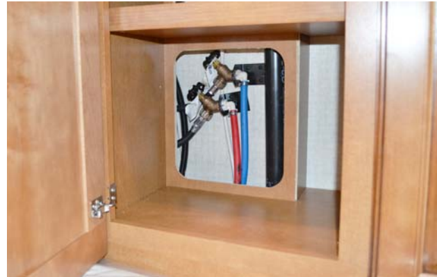
Water Supply Faucets (Located inside cabinet front of washer/dryer - remove access panel) *Model 35F shown
