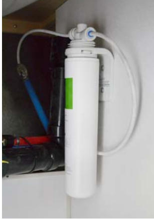
Ice Maker Filter Assembly (Located below galley sink) -Typical Installation
