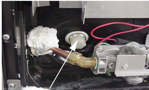
Water Heater Drain Plug (Remove with socket)
