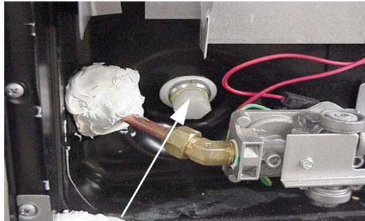
Water Heater Drain Plug (Remove with socket)
