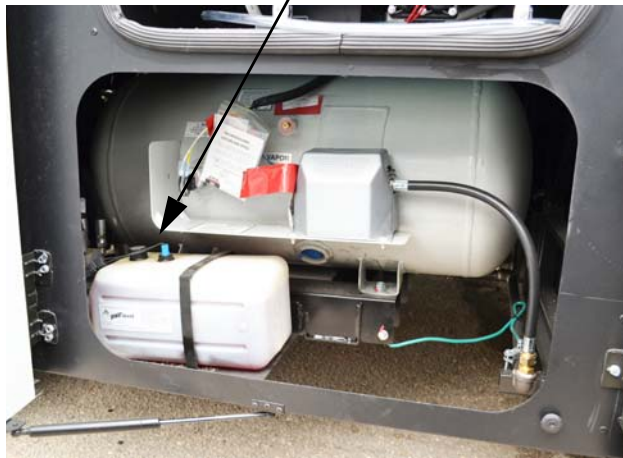
Hydraulic Oil Reservoir (Located inside left exterior compartment behind front tire) -Typical View
