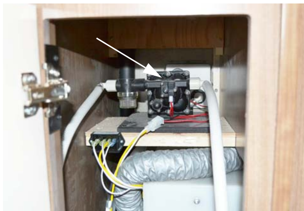
Water Pump (Located beneath removable access panel in pantry) -Model 23B shown
