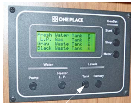
Tank Levels Switch
