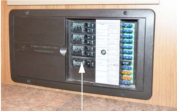
120-Volt Circuit Breakers -Typical View
