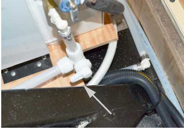
Water Heater Bypass Valve -Typical installation shown
