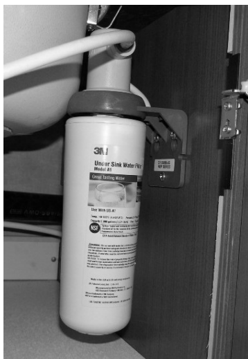
Cold Water Filter Assembly (Located below galley sink) NOTE: Hot waterline is not filtered.
