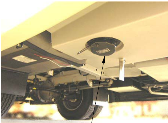
Sewage Drain Outlet (Located on the underside of water service center) -Typical View
