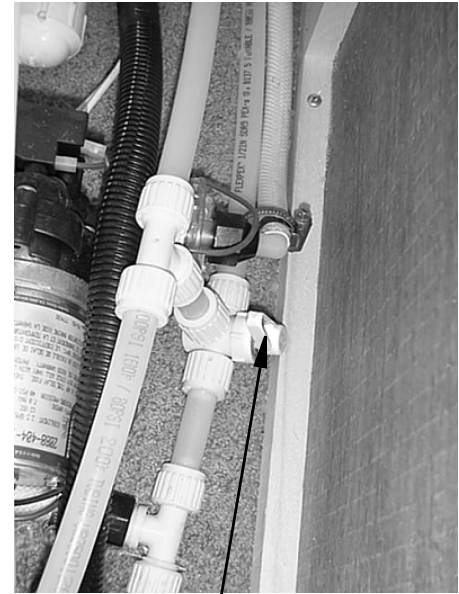
Waterline Drain Valve (Typical)
