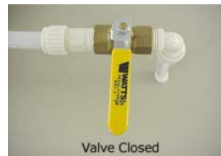
Water Tank Drain Valve (Typical)
