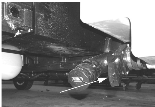
Black Waste Tank Drain Valve (Located beneath coach on mid-driver side) -Typical View
