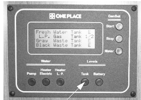
Tank Levels Switch
