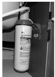
Cold Water Filter Assembly (Located below galley sink) NOTE: Hot waterline is <u>not</u> filtered.
