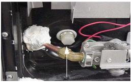
Water Heater Drain Plug (Remove with socket)
