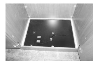
3. Rotate the Locking Arm fully CLOCKWISE to the **locked** position, securing the Wardrobe Cabinet to the floor plate.
