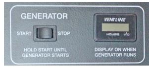
Generator Switch and Hourmeter on monitor panel
