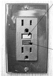
GFCI Outlet (Ground Fault Protector)
