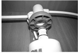
• Insert new filter up into filter socket - press and twist 1/4 turn "clockwise".
