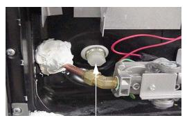
Water Heater Drain Plug (Remove with socket)
