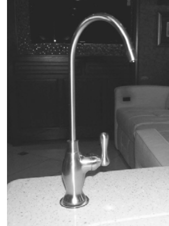
Filtered Water Faucet -Typical View
