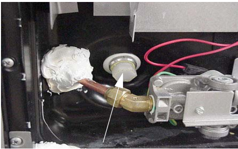
Water Heater Drain Plug (Remove with socket)
