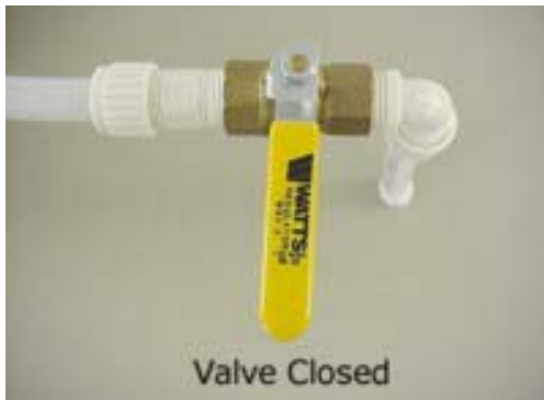
Water Tank Drain Valve -Typical installation shown
