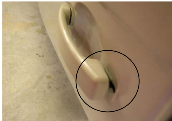
Door Unlatched (note gap)
