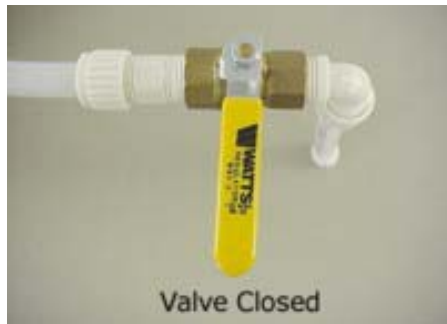
Water Tank Drain Valve (Typical)
