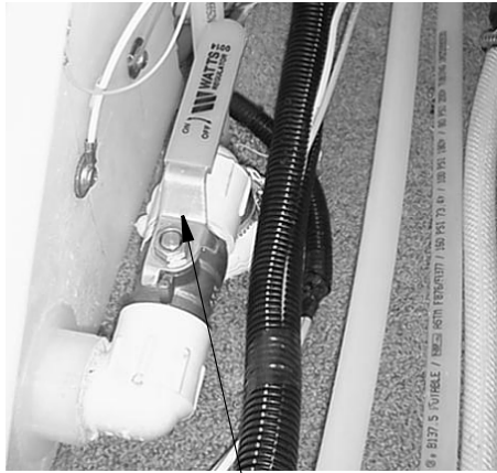
Water Tank Drain Valve (Typical)
