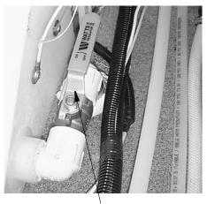
Water Tank Drain Valve (Typical)
