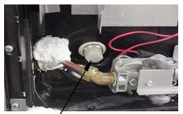
Water Heater Drain Plug (Remove with socket)
