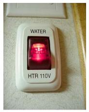
Electric Water Heater Switch (Typically located near Systems Monitor Panel)
