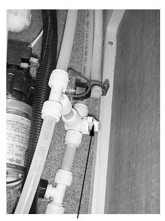
Waterline Drain Valve (Typical)
