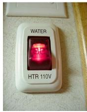
Electric Water Heater Switch (Typically located near Systems Monitor Panel)
