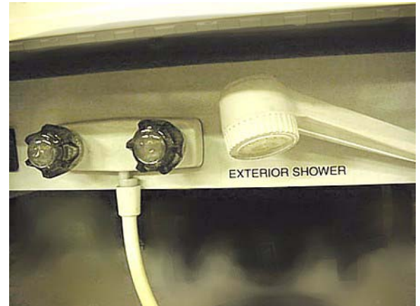
Exterior Shower/Wash Station -Typical View
