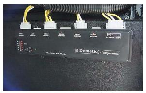
Awning Control Box (Located in exterior compartment)
