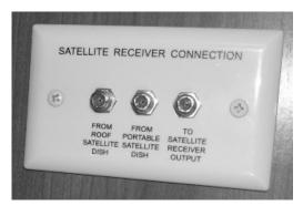
Interior Connection for Satellite Dishes (Located in cabinet near TV) - Typical View
