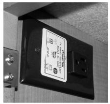
Front TV/Buffet TV Ignition Switch Interlock -Typical View
