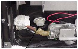
Water Heater Drain Plug Remove with socket
