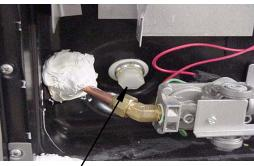
Water Heater Drain Plug Remove with socket
