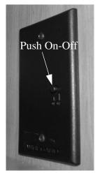
TV Signal Amplifier Switch inside overhead cabinet near TV (Typical View) -Model J37F shown
