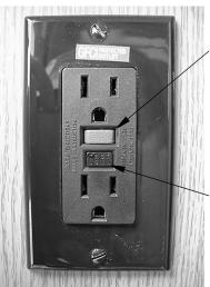
GFCI Outlet (Ground Fault Protector) Push to Reset circuit after monthly testing or ground fault tripping.
