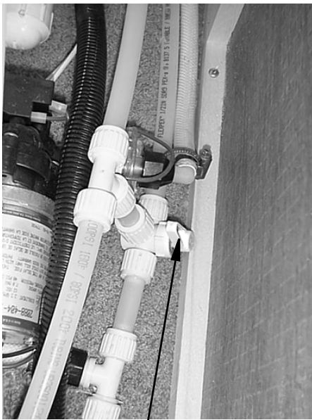
Waterline Drain Valve (Typical)
