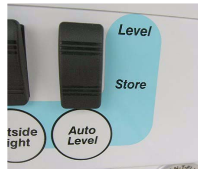
Auto Level Switch in Service Center Compartment (Typical View)
