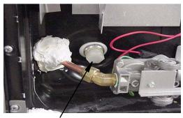
Water Heater Drain Plug Remove with socket
