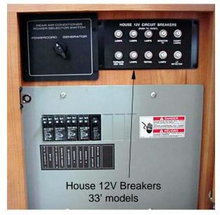
A label on the panel states the amperage rating and circuit protected for each fuse or breaker.
