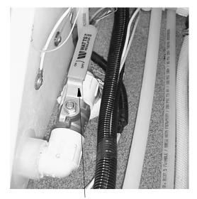
Water Tank Drain Valve (Typical)
