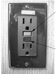
Push to Reset circuit after monthly testing or ground fault tripping.
