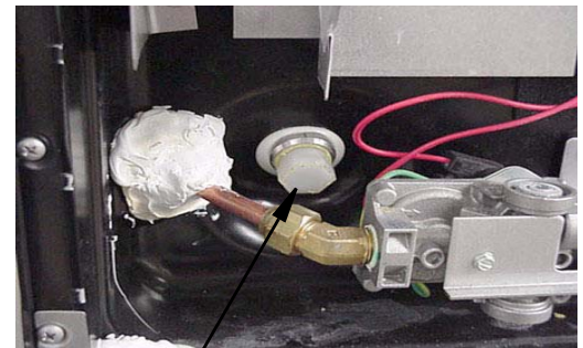
Water Heater Drain Plug Remove with socket
