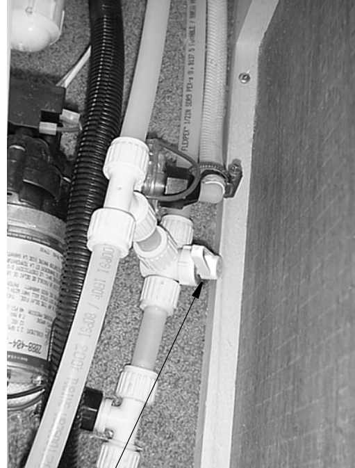
Water Heater Bypass Valve (Typical)
