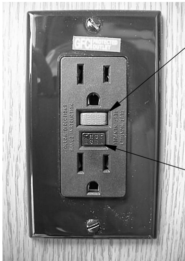
GFCI Outlet (Ground Fault Protector)
