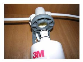
• Install the diverter plug into the filter socket. Insert plug up into the filter socket as far as possible and twist clockwise (to the right) one-quarter turn until it stops.
