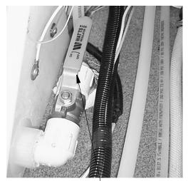
Water Tank Drain Valve (Typical)
