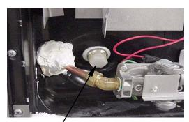
Water Heater Drain Plug Remove with socket.
