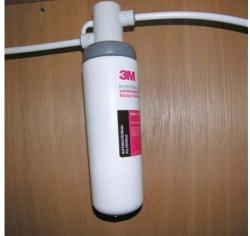
Cold Water Filter Assembly below Galley Sink (Hot water line is not filtered.)
