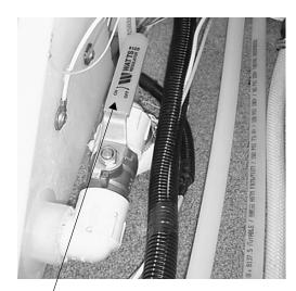
Water Tank Drain Valve
