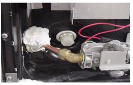
Also open the Pressure-Temperature relief valve at the top right portion of the tank to prevent air locking in the tank while draining.
