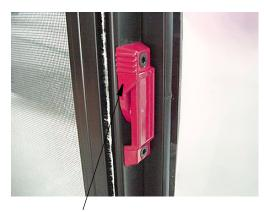
Pull latch outward to slide window open
