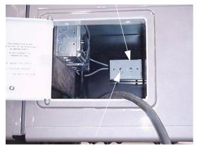
Portable Satellite Dish Hook-up in Shoreline Compartment
