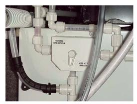
Water Heater By-Pass Valve (Typical)
