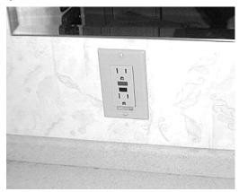
Ground Fault Circuit Interrupter (GFCI)
