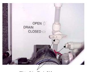
Water Line Drain Valves (in water pump compartment)
