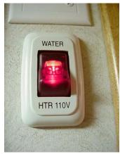
Electric Water Heater Switch (Typical)
