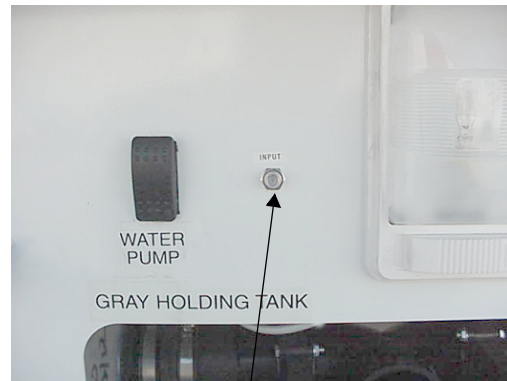
Cable TV Hook-Up in Utility Compartment
