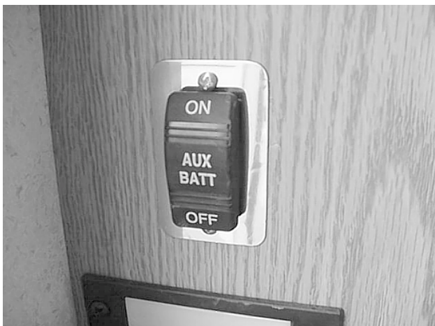
Aux. Batt. Switch (Near entrance door)
