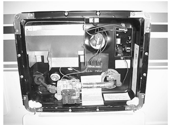
Water Heater Exterior Service Access
