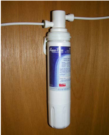
Filtered Water Faucet/Ice Maker Filter Assembly (Located below galley sink)
