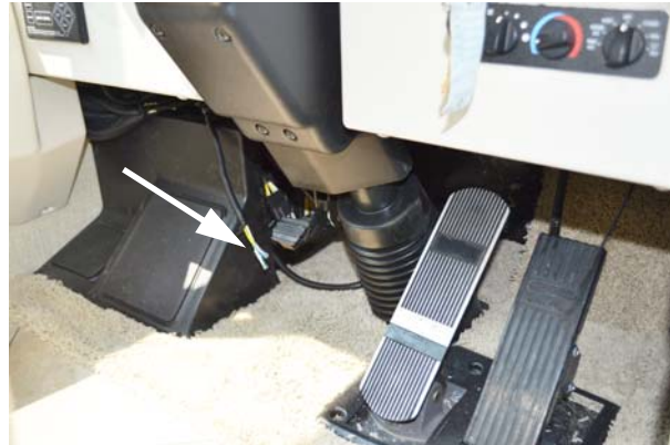
CB Power Wires -Typical View
