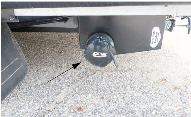
Sewage Drain Outlet (Located beneath motorhome) *Model 59KL -Typical View
