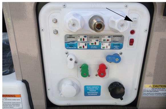
Pump switch -Typical View
