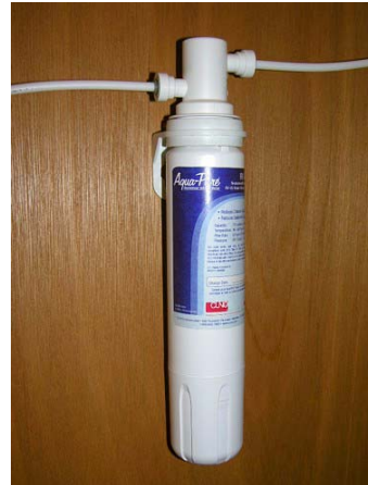
Water Filter Assembly below Galley Sink
