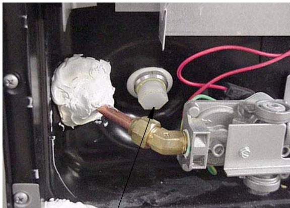
Drain Plug Water Heater Service Access
