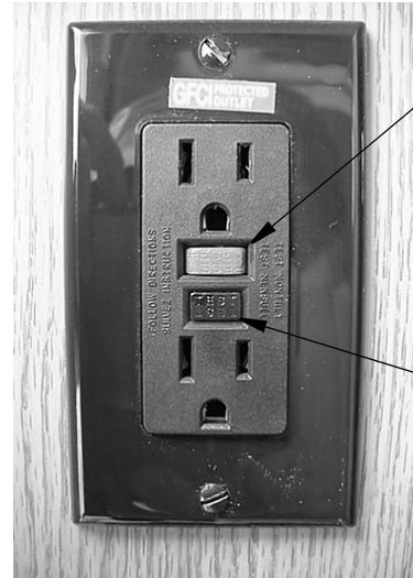
GFCI Outlet (Ground Fault Protector)
