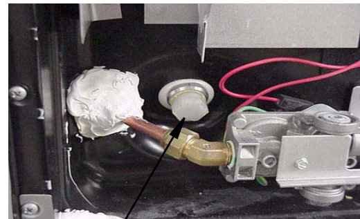
Water Heater Drain Plug Remove with socket
