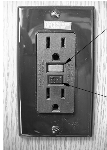
GFCI Outlet (Ground Fault Protector)
