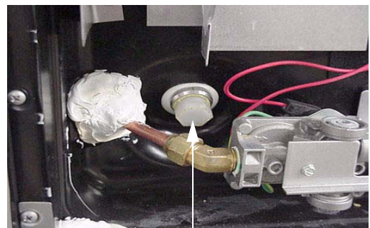
Water Heater Drain Plug (Remove with socket)
