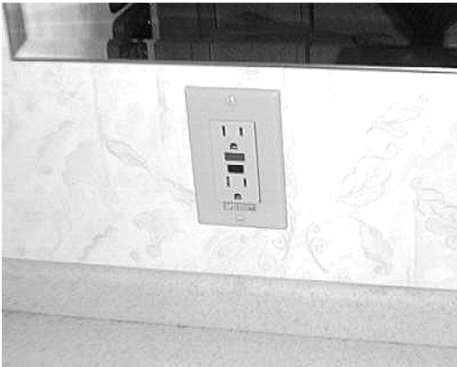
Ground Fault Circuit Interrupter (GFCI)
