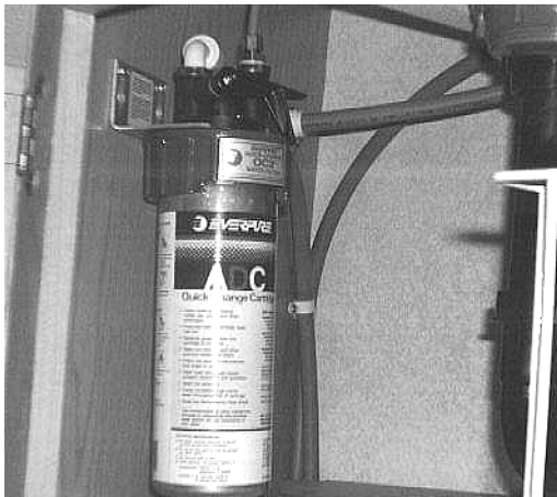
Water Filter Assembly - Below Galley Sink
