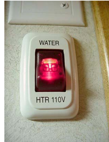
Electric Water Heater Switch (Typical)
