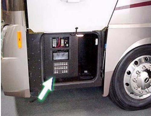
12V Electrical Compartment
