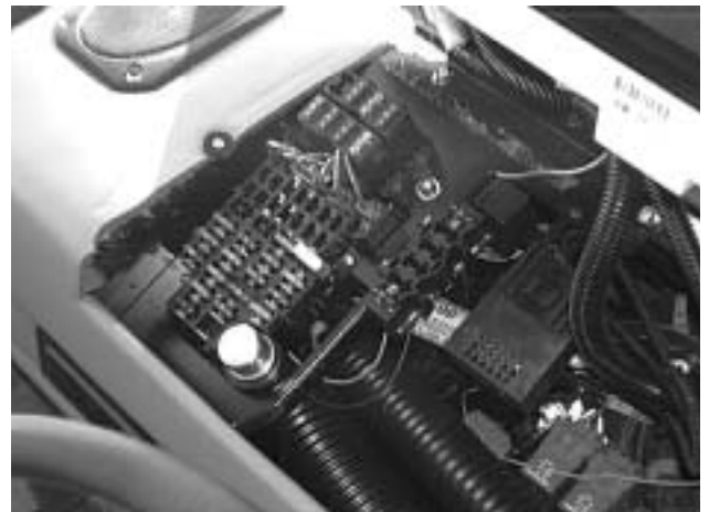
Automotive 12-Volt Fuse Block (under dash pad - lift up)
