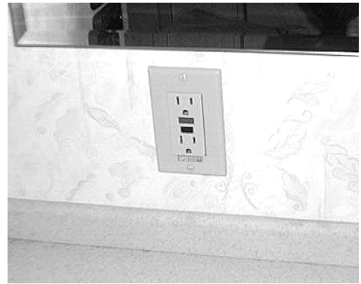
Ground Fault Circuit Interrupter (GFCI)
