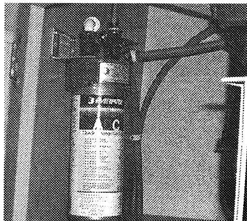
Water Filter Assembly - Below Galley Sink
