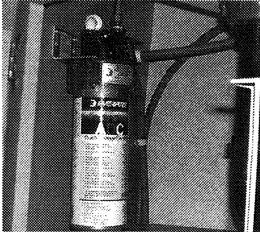
Water Filter Assembly - Below Galley Sink
