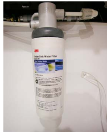
Galley Filtered Cold Water Faucet/ Ice Maker Filter Assembly (Located below galley sink) -Typical View
