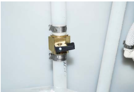
Water Tank Drain Valve -Typical installation shown
